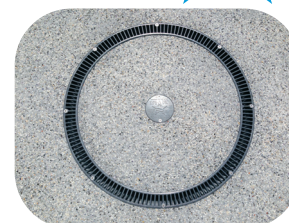
Top view of completed Full Circle® drain
