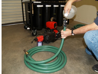
Fill hose with water
