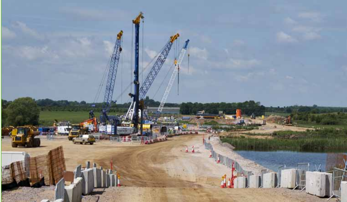
Work on the River Great Ouse Viaduct is progressing well
