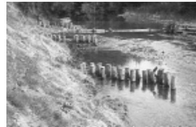
*Seek expert advice if installing bank stabilisation structures such as pin groynes*
