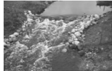
*Seek expert advice if installing bed control structures such as rock chutes*
