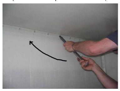
Recommended direction of Lock Pin removal: Parallel to line of fasteners as shown.
