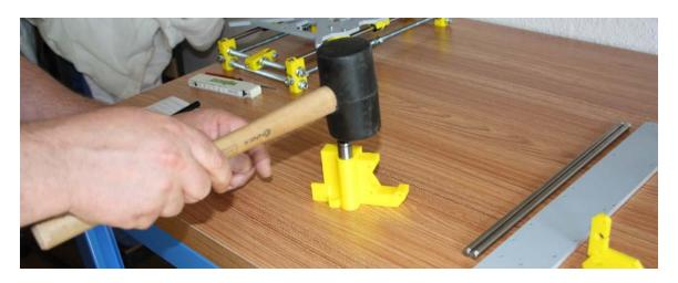
Push two LM8UU bearings in the X End Idler, and two LM8UU bearings in the X End Motor parts. Use a rubber mallet for this procedure.
